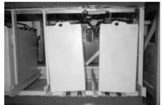
This photo shows an actual slide strip installation, note that the batteries are leaning against the uprights.
